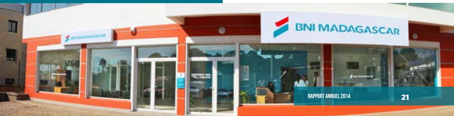
Facade Agence Ivandry
